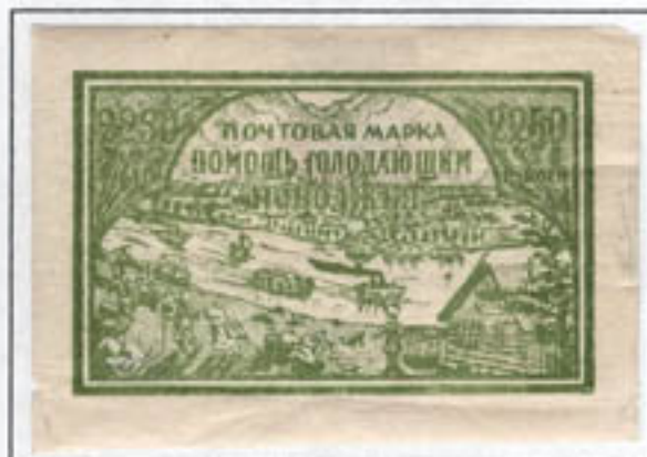
Relief work on Volga River
