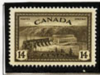
HYDROELECTRIC STATION, ST. MAURICE RIVER
