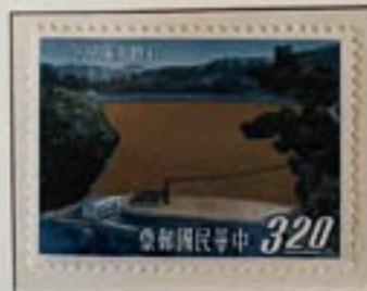
Dam and Powerhouse
